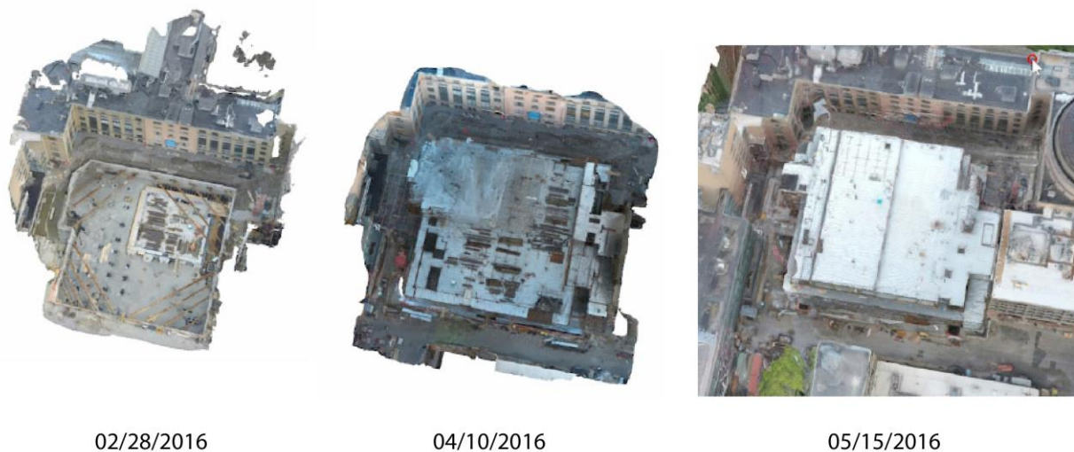
Figure 8. Comparative viewing of the MIT Nano building construction site captured in different months.
